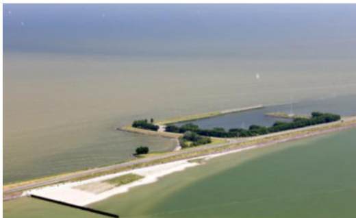
Houtrib Dike Pilot Project
